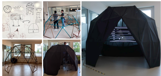
Figure 3. The images show the construction of the dome, from sketches and assembling to placing the custom-shaped black fabric to create a dedicated dimly lit space for interaction.
